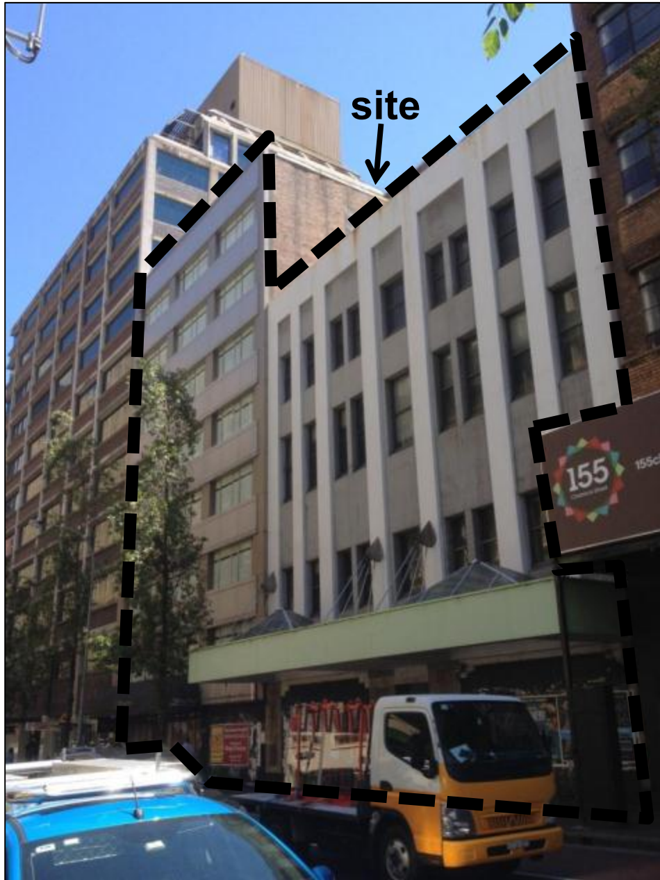
Figure 2: The existing buildings on site as viewed from Clarence Street
